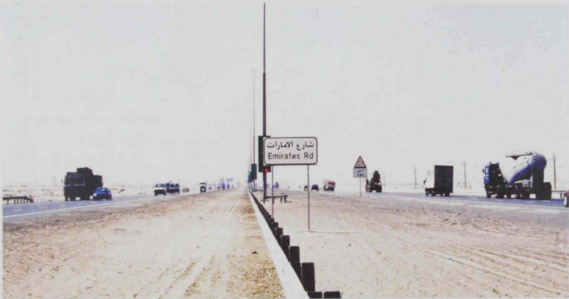
Figure 4-20: Emirates road is one of the most significant changes that has happened in Dubai area during the time between 1993 & 2000. The road starts from Jebel Ali area and finishes in the border of Sharjah City.
