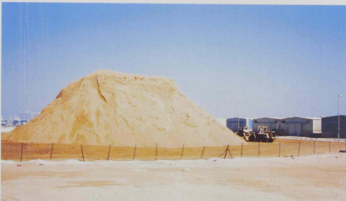
Figure 4-29: Huge amount of earth have been moved and transported to reclaim land from the sea in many parts of Abu Dhabi coastal area. The photo is showing an example of a huge pile of earth which is ready to use for reclamation purposes.
