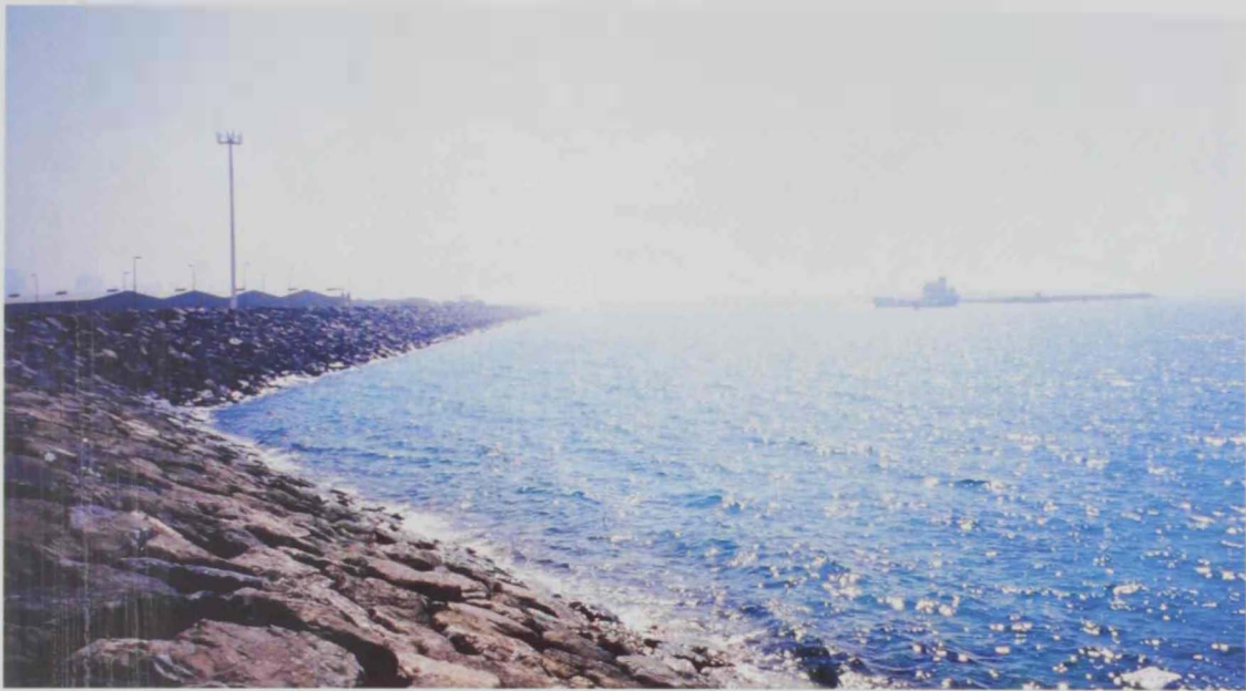
Figure 4-4: Large and long sea breaker has been created in Zayed Port for protection from sea waves. The photo is showing the main sea breaker in Zayed Port.
