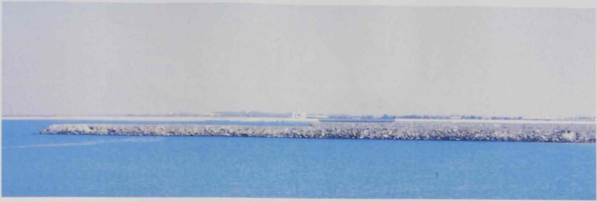
Figure 4-9: This is an example of sea breakers along Al Raha Beach. It consists of hard igneous rocks that were delivered from the northern emirates mountains.
